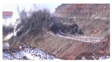
DIFFERENTIAL ENERGY technology allowed the operators to adjust the explosive energy in each hole based on the geology.
